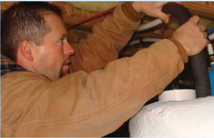
South River EMC Energy Specialist Robby Talton fits pipe insulation.
