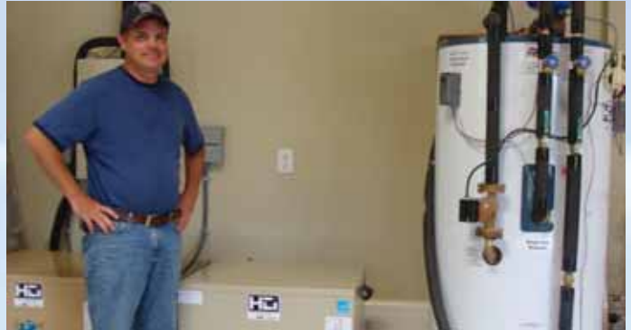
Wayne Underwood with his geothermal units and water heater.
