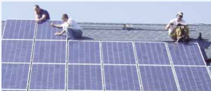
AEC employees work to install a photovoltaic unit on a home.
