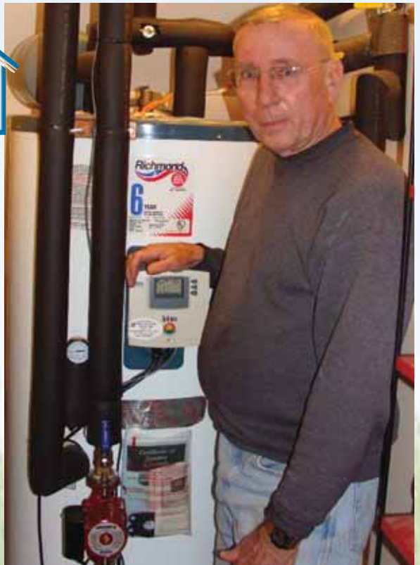
Member Frank Stump installed an 80-gallon solar water heater with an electric back up.
